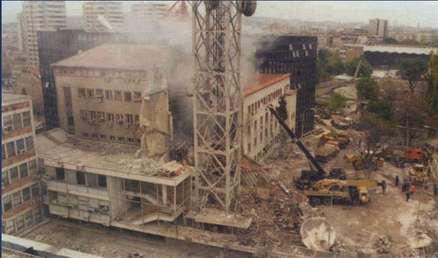
Photo 33 Broad view of demolished RTS office building at 1 Aberdareva Street 23 April 1999
